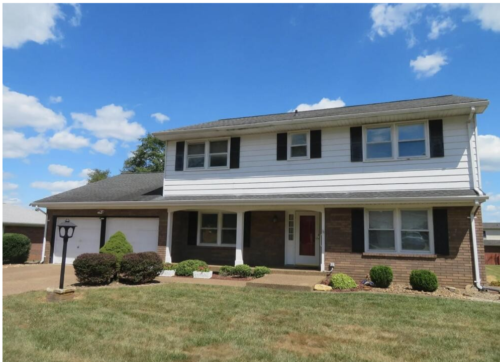
Photo A-1: Exterior front – Example SFR (address omitted)
